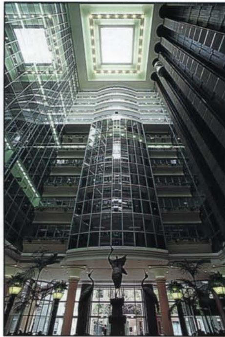
In addition to the Atrium ceiling, Geelong Fabrications provided steelwork for the main tower roof, gallery walkways, Atrium pyramid and shop fronts at 530 Collins Street.
