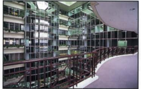
Steelwork for the Atrium ceiling at 530 Collins Street was erected for 14 floors without scaffolding.
