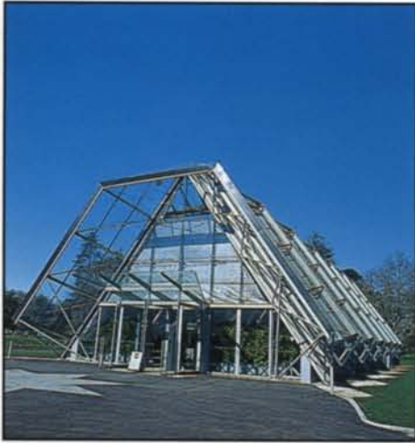
Plane trussing was introduced to enhance the structure's stiffness and improve efficiency by reducing and increasing flexural and axial loads respectively.
